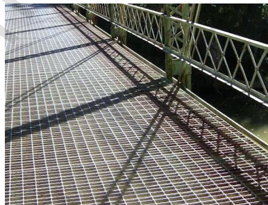
Steel grating bridge decks
