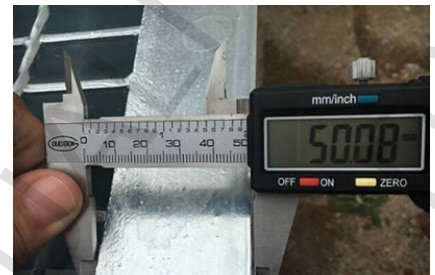
Angle bar size inspection
